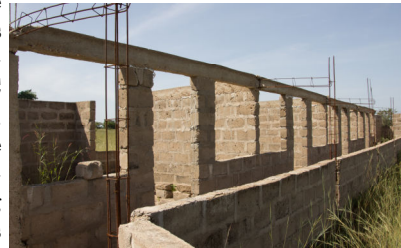
Our new home is taking shape
